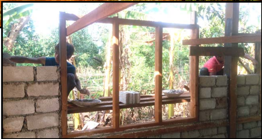
Replacing the walls at the Namhu mission station
